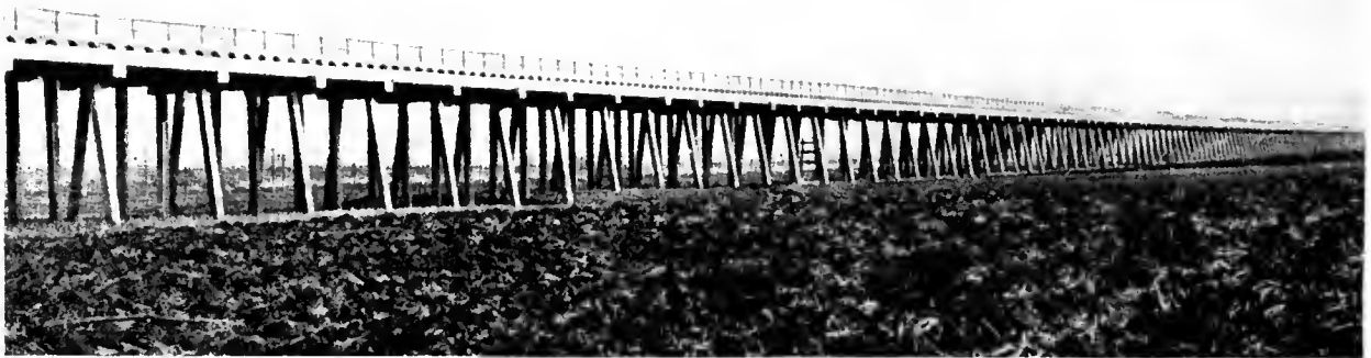
Reinforced concrete highway trestle 3\frac{1}{4} miles long over Yolo By-Pass, California.
